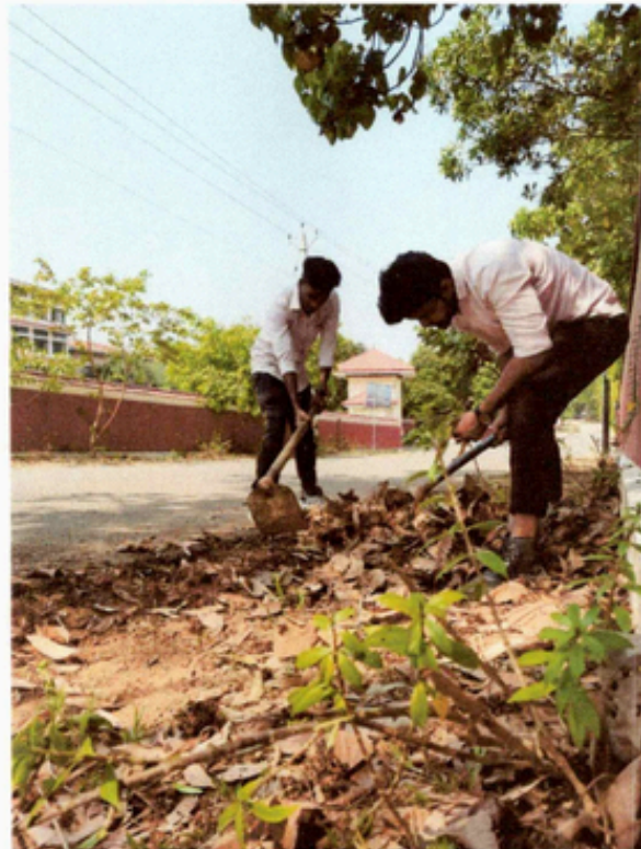
Cleaning of engineering college road
