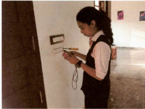
Electrical damage repair
